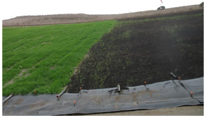
November 13: In area of compost application on the right, seedlings are just beginning to emerge; hydroseeded area, on the left, where seed was applied two weeks earlier, up and growing.
